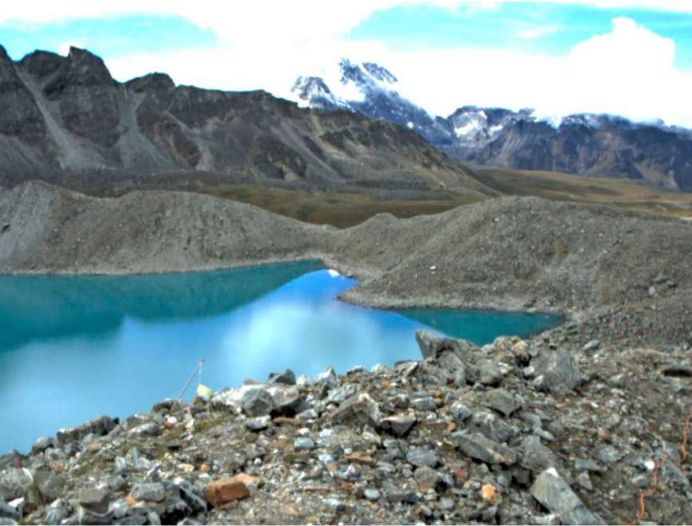
Definite risk: The south-end of the Shako Cho lake (5,200 m) in north Sikkim. The south-end shows the weak debris that forms its moraine-dam. NDMA
